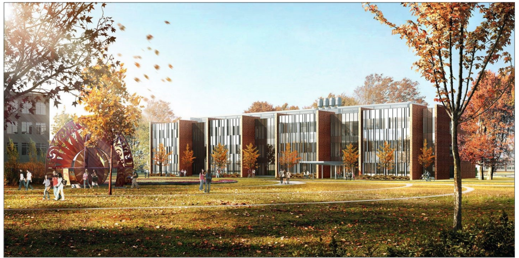
Flex Labs building where the Purdue CISTAR laboratories are located
