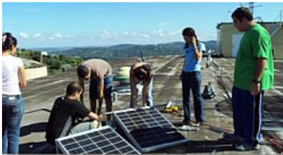
Student researchers in Mayaguez, Puerto Rico installing solar panels to power their OTG radar system.
